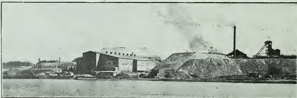
AIR COMPRESSOR STATION, VICTORIA FALLS AND TRANSVAAL POWER COMPANY.
